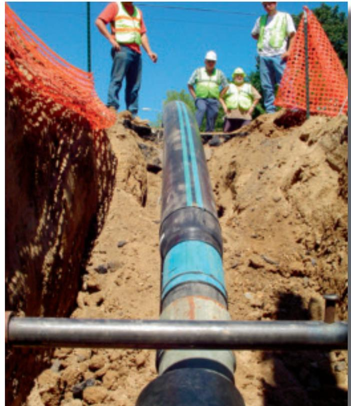
*One section of the 1,600 total linear feet of 14-inch high-density polyethylene (HDPE) pipe is lowered into the ground. It was the first time in Lansing's history that both HDPE pipe and pipe bursting were utilized.*
