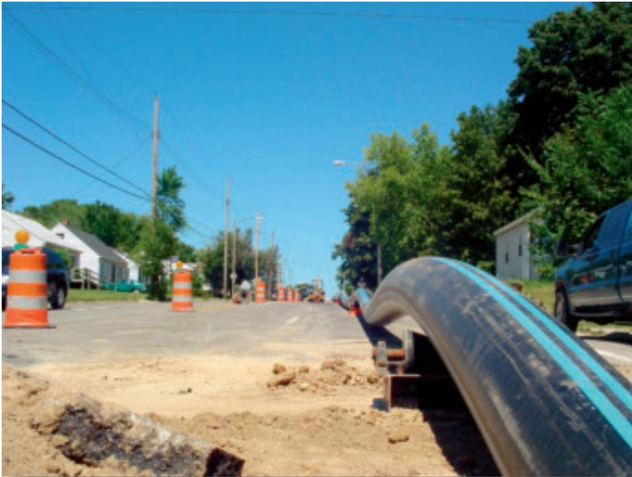
City engineers estimated that using HDPE pipe meant the project was completed in about 60 percent of the time it would have taken with traditional excavating. Moreover, the resulting re-paving was completed with just two inches of asphalt instead of 10 inches of concrete and four inches of asphalt, due to almost no ground disruption.
